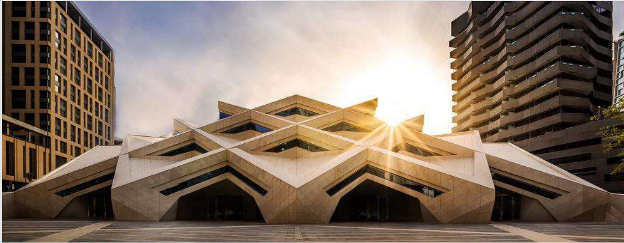
KAFD Mosque, Saudi Arabia
