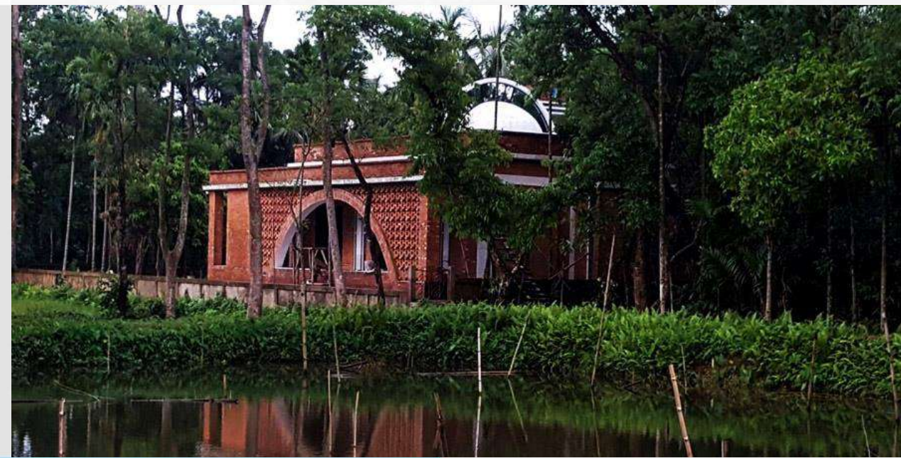
Teradol Community Mosque , Bangladesh
