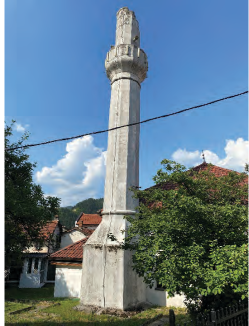
Figure 15 : Minaret of the Vardačka mosque of Konjic (central Herzegovina), with its upper part and roof still missing, since they were destroyed by shelling.
