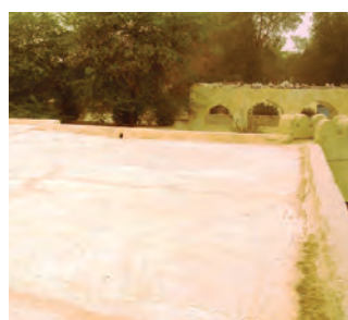
Figure 21. Roof slab is covered with earth plaster. Source: Author.
