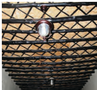
Figure 20. False Ceiling made out of tree branches and reeds.
