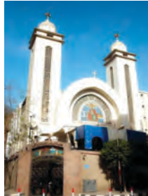
Saint Mark in Minyat al-Sirg.(1960) Largest Church
