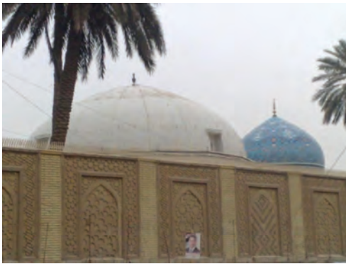
P7: Al-Jailany Mosque Eastern elevation
