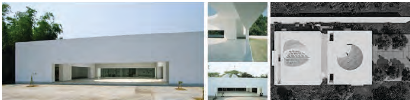
Fig. 10: Chandgaon Mosque, Chittagong, Bangladesh is a bold statement of an Emerged Mosque architecture.
