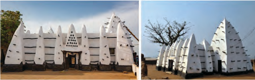
Fig. 8: The restored and conserved Larabanga Mosque in Ghana as a clear example of Vernacular Architecture.
