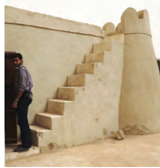
Figure 18. The southern bastion accessed by steps. Source: Author
