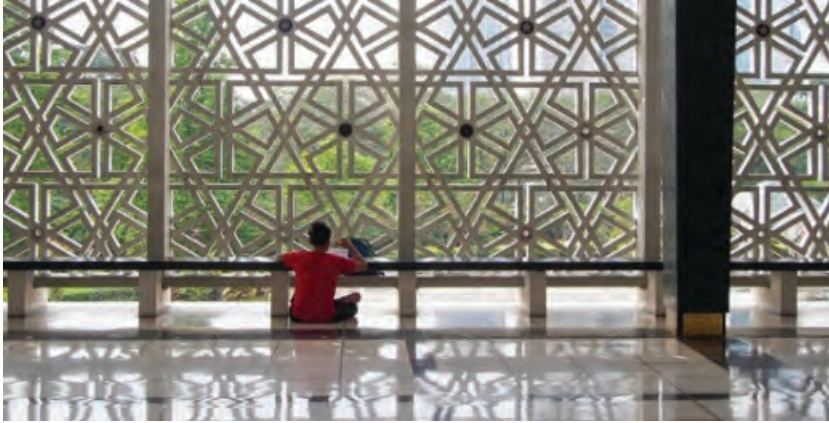
Figure 6: Ornamentation of the screen wall from the veranda area of National Mosque has function as ventilation and also natural lighting to the space. Source: www.pixshark.com
