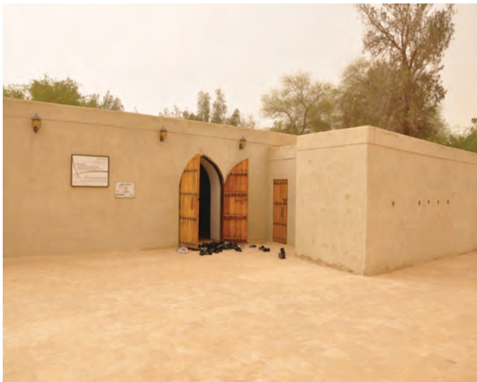
Figure 14. Exterior of the west entrance. Source: Author
