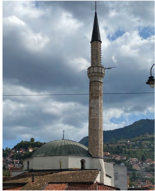
Figure 2 : Minaret of the Čekrekčijina mosque (Sarajevo), with the base of its kaca nested within the cupola.
