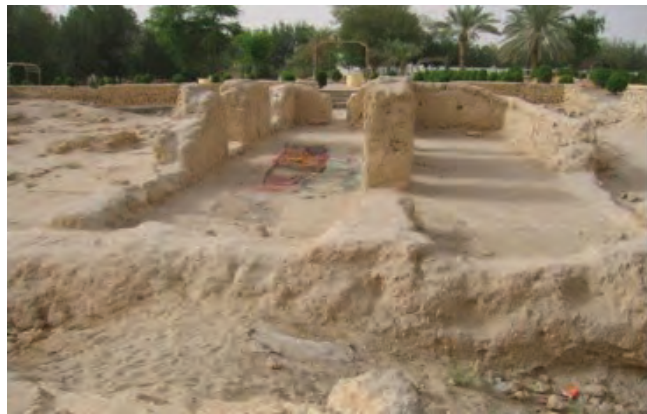
Figure 4. The earth walls of Jawatha Mosque ruin before restoration. Source: Al-Moghanam, 2006.
